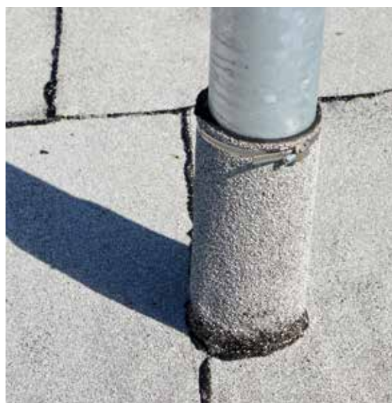
Obr. 2 – Detail, oprava prostupu
